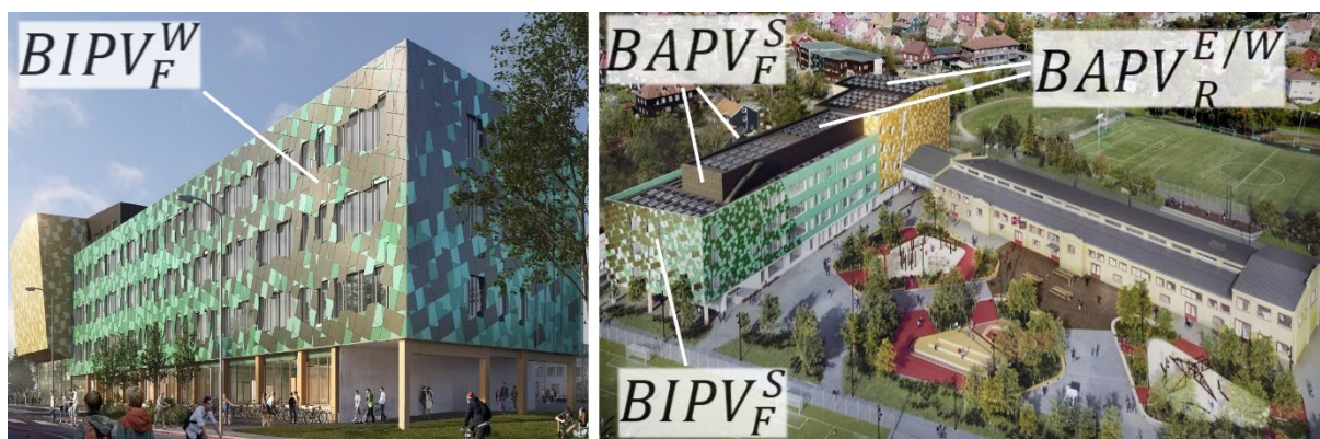
Figure 1. View of the S-building west façade (left) and overview of the ARV pilot Voldsløkka school with PV systems on the roofs and facades (right): Image courtesy of Veidekke.
